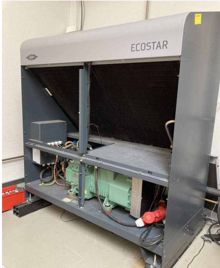
Ecostar is a condensing unit for supermarket refrigeration systems
